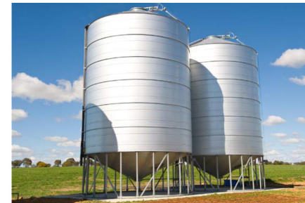
Figure 2.3.9 Dry Silo Storage
